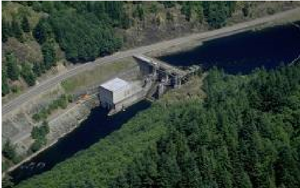
Figure 6. Photograph showing Big Cliff Dam on the North Santiam River, Oregon. Photograph by the U.S. Army Corps of Engineers.
