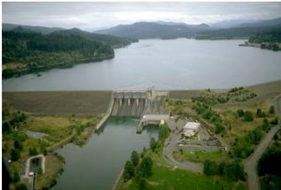
Figure 19. Photograph showing Foster Dam on the South Santiam River, Oregon. Photograph by the U.S. Army Corps of Engineers.
