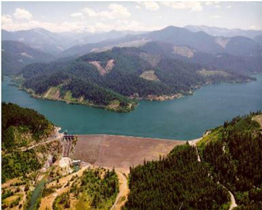
Figure 37. Photograph showing Hills Creek Dam and Hills Creek Reservoir on the Middle Fork Willamette River, Oregon. Photograph by the U.S. Army Corps of Engineers.
