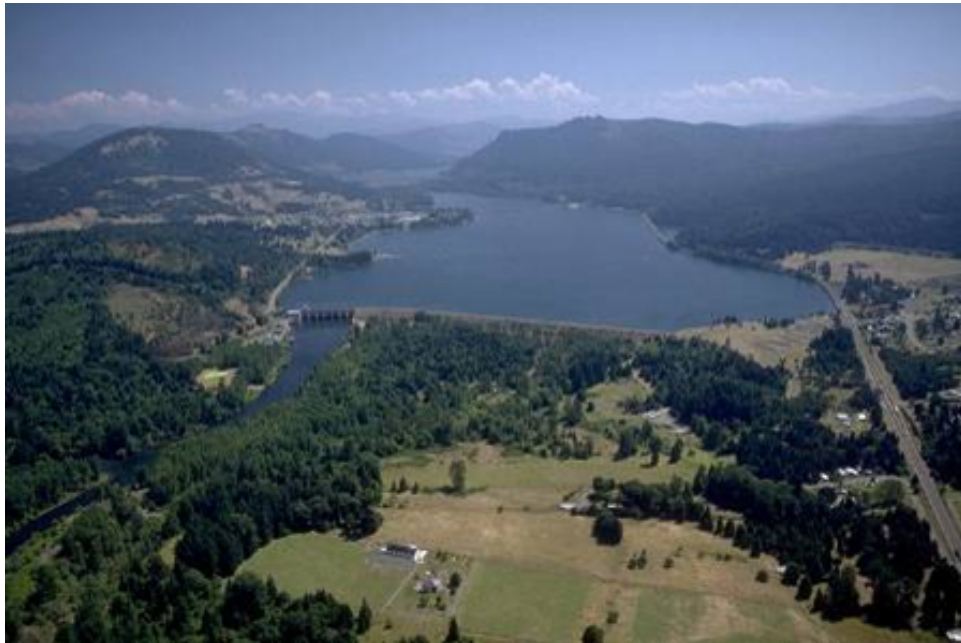
Figure 40. Photograph showing Dexter Dam and Dexter Reservoir on the Middle Fork Willamette River, Oregon. Photograph by the U.S. Army Corps of Engineers.
